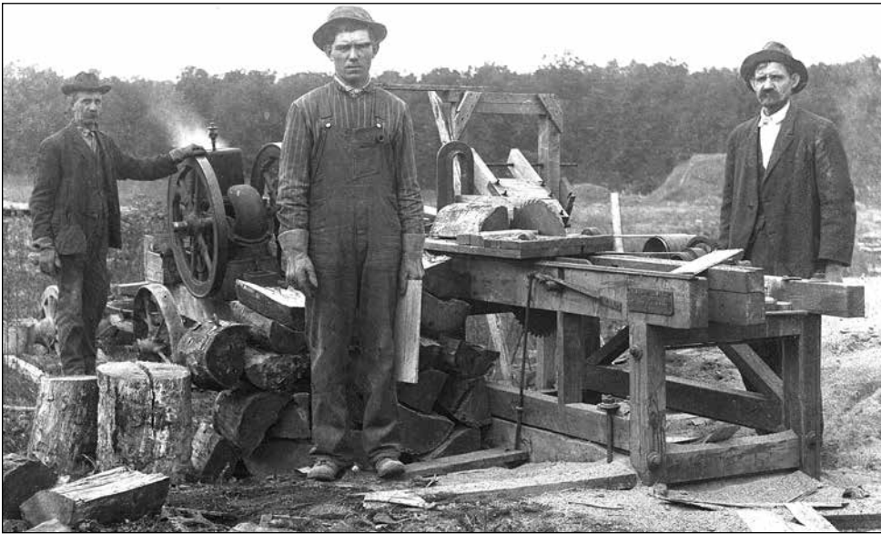
Gasoline-powered shingle saw mill
